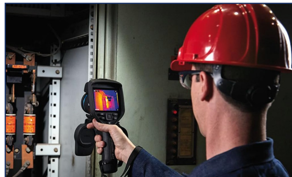
Thermographic infrared heat scanning
