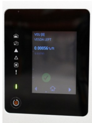
VESDA continuous air sampling smoke detection
