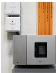
VESDA continuous air sampling smoke detection
